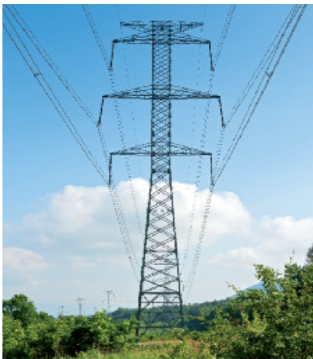
Soudek - nosný (2x400 kV) Barrel tower - Suspension tower (2x400kV)
