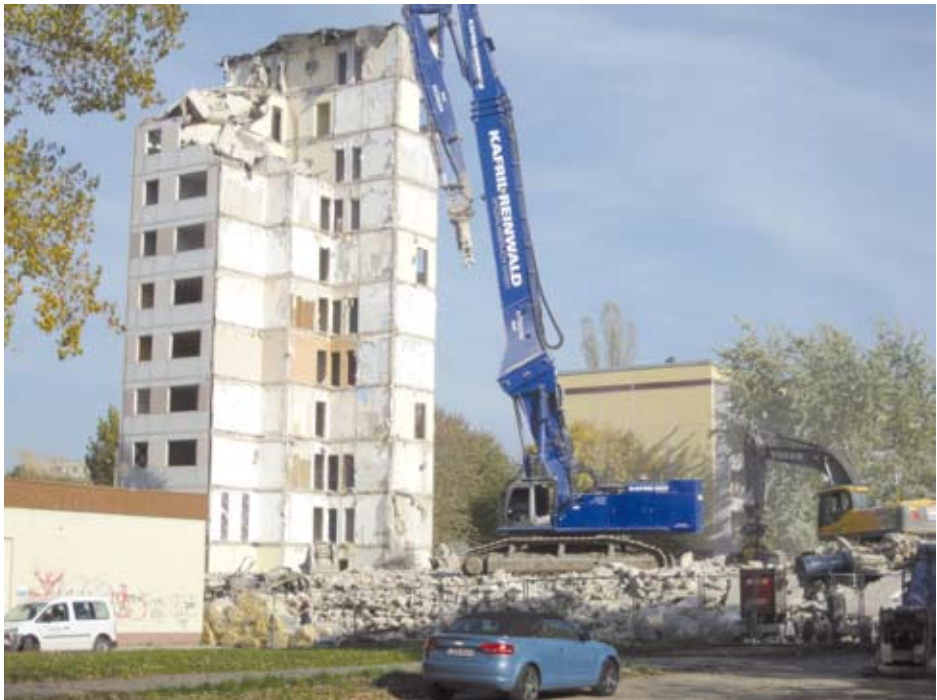
Figure 1 Demolition of empty prefabricated houses in Halle Neustadt 10
